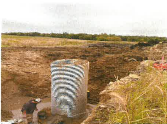
Installation of the agridrain.
