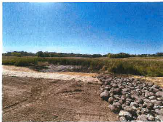
Completed berm and spillway.
