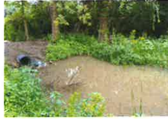
Completed sediment basin
