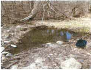
Erosion coming from neighboring parcel
