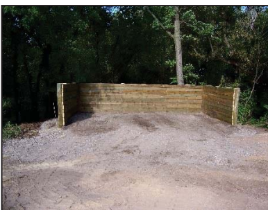
After: Manure, bedding and nutrients contained, easier to access, better compost; nutrients conserved, runoff pollution curtailed; cleaner water.
