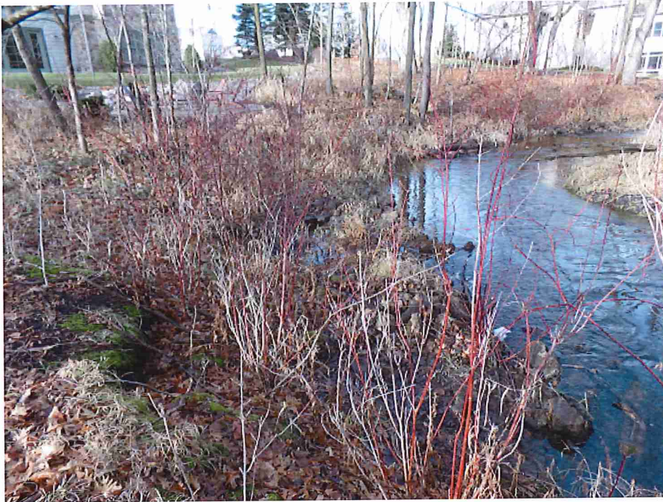
Stream Barbs and Shrubs from 2006 project still functioning to protect slopes along Rush Creek (photo December 2015).
