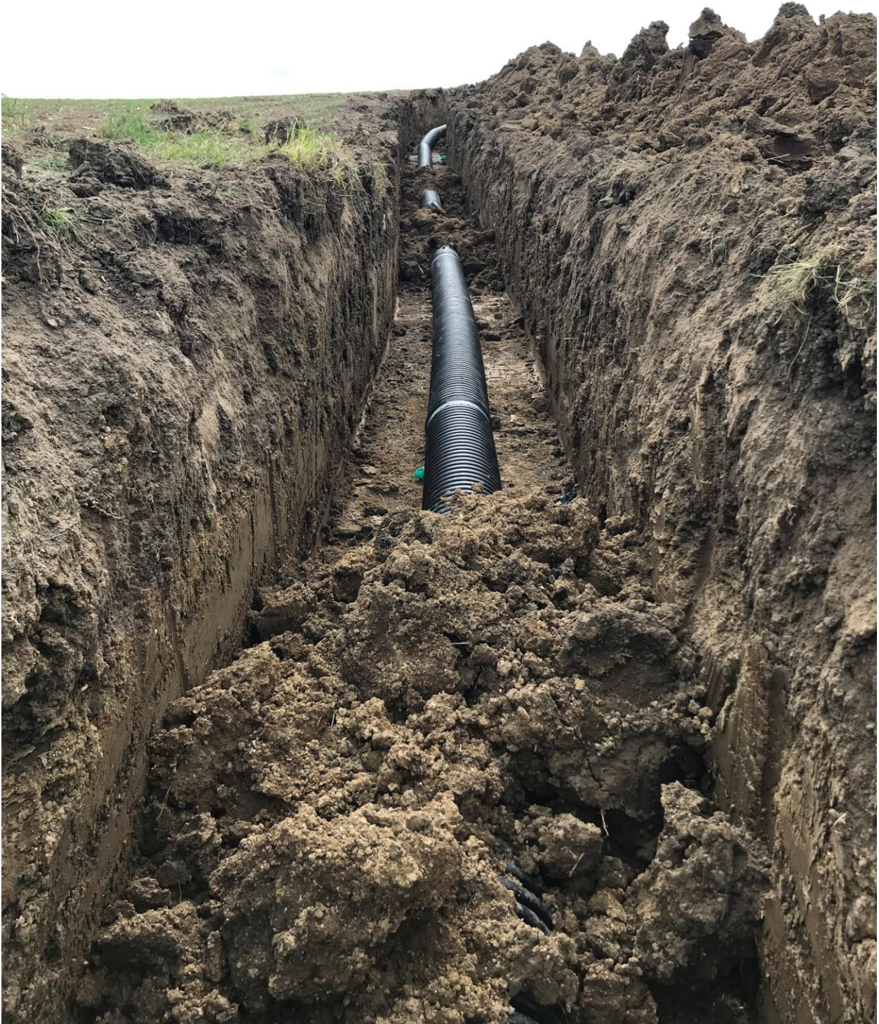
Figure 1: Top of Hill Waterway Pipe Installation
