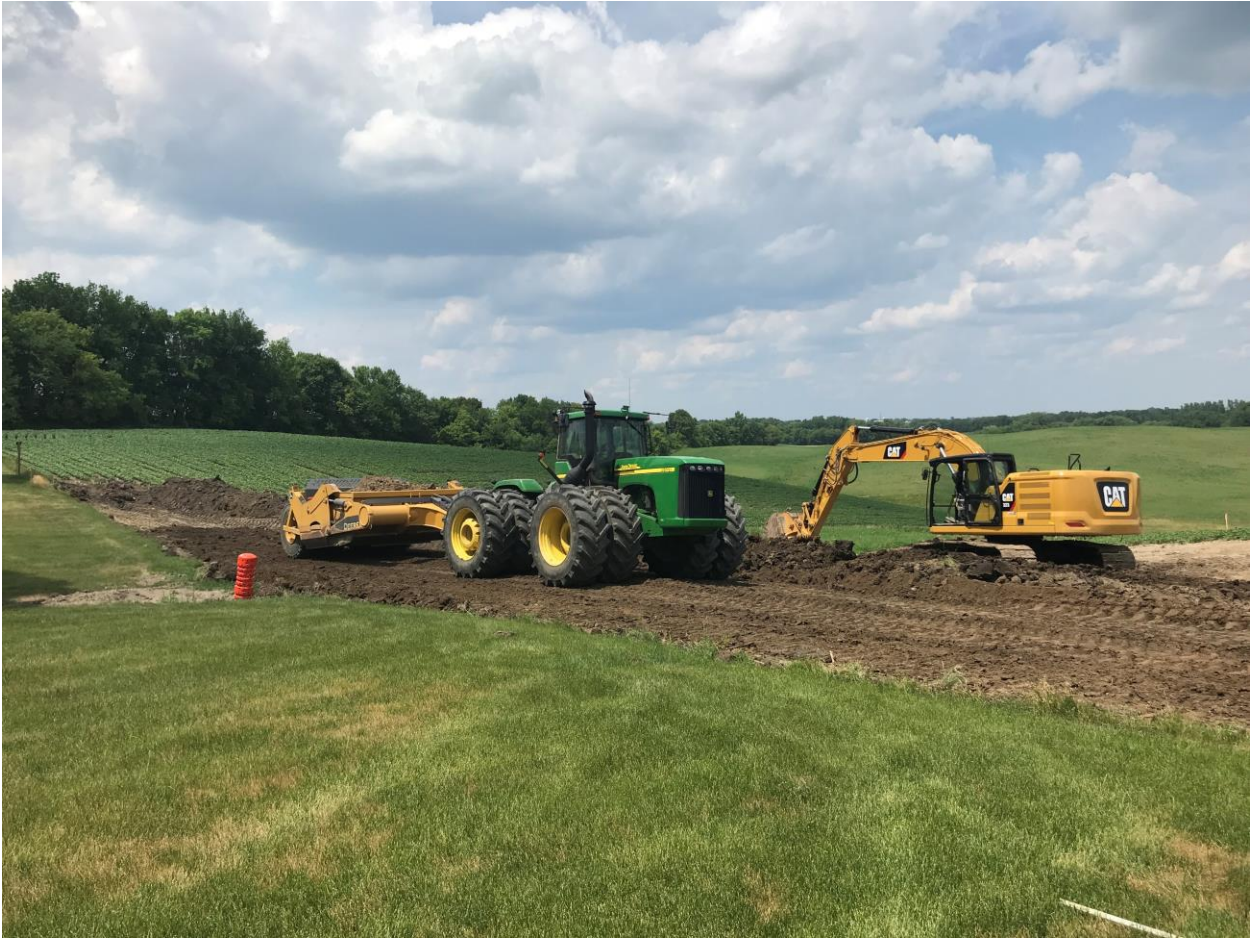
Figure 4: WASCOB Construction
